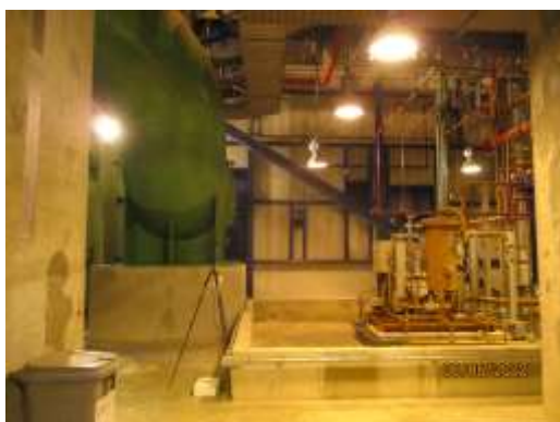
Steam Turbine Lube Oil Skid Block 2
