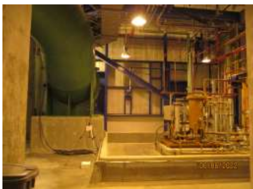
Steam Turbine Lube Oil Skid Block 1
